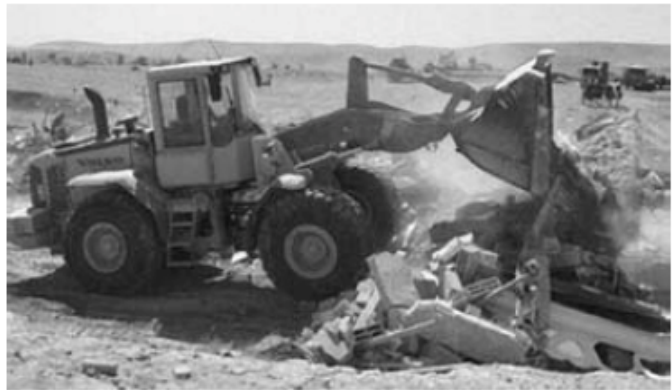
Destroying Bedouin home in the Negev
